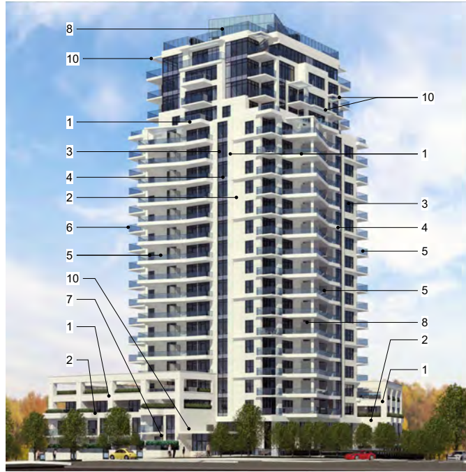
PREFINISHED ALUMINUM WINDOW FRAME (FOR # 3 & 4) (CHARCOAL GREY)
