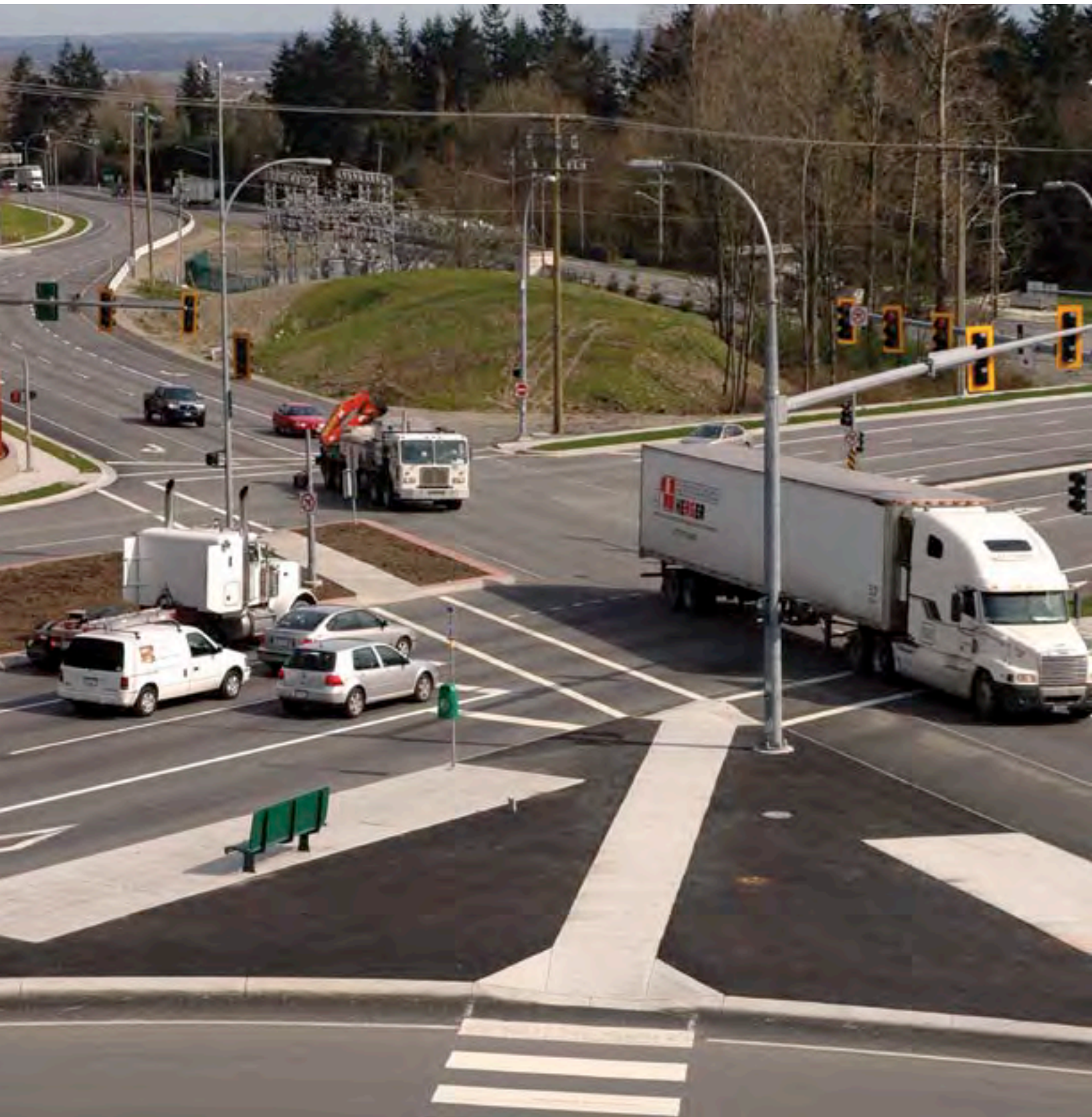
King George Highway Upgrades
