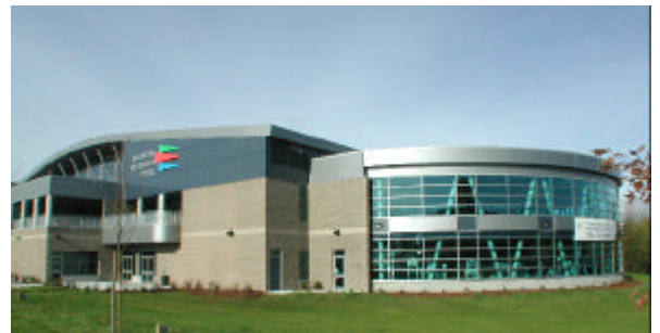
Figure 1 - Guildford Recreation Centre
