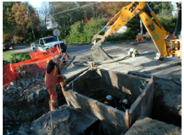
Figure 1 - Drainage work in South Surrey
