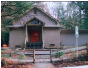
Figure 2 - Elgin School Before Restoration
