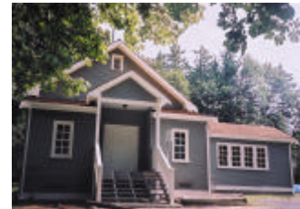
Figure 3 - Elgin School After Restoration
