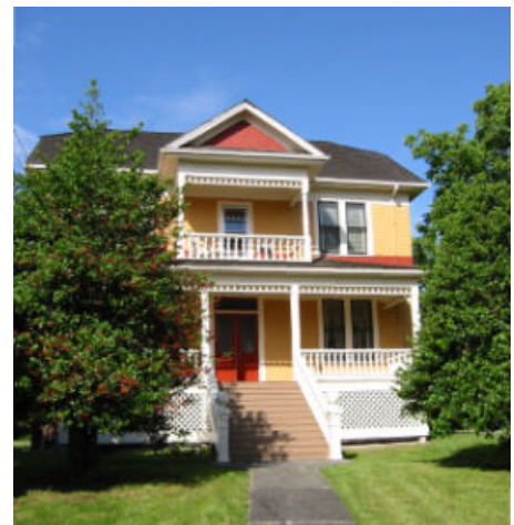
Pilath Hall Heritage Building
