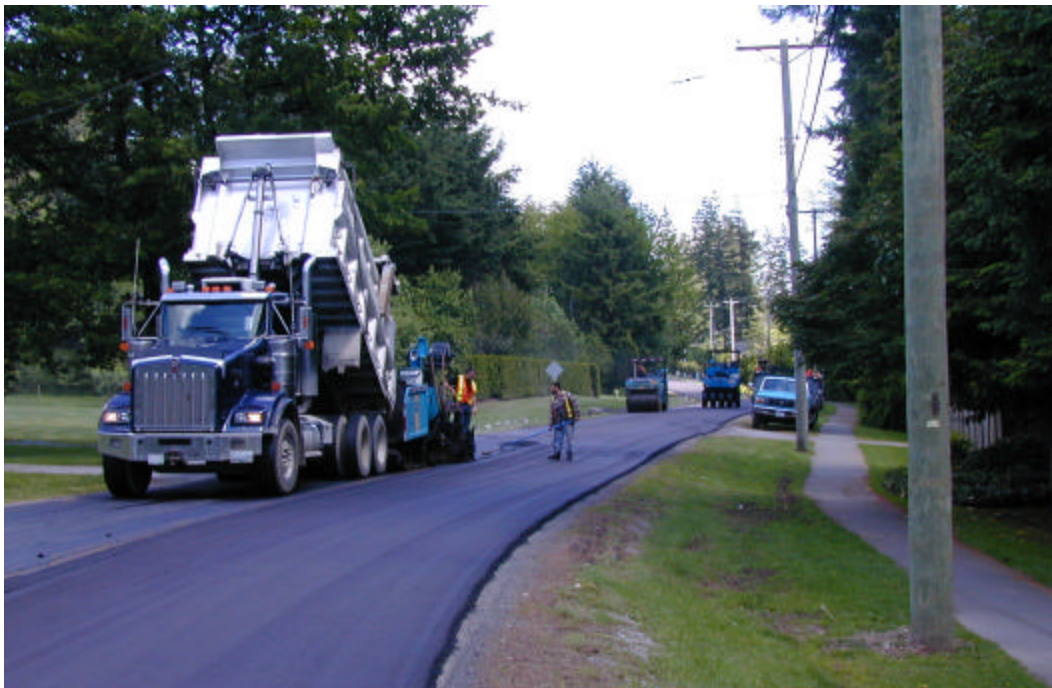
New McLellan Road Work
