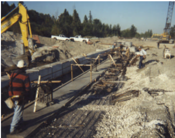
Scott Road Improvements
