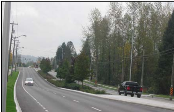
Upgraded Section of Fraser Highway
