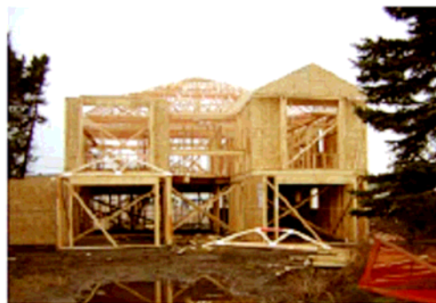
Single Family Dwelling Under Construction
