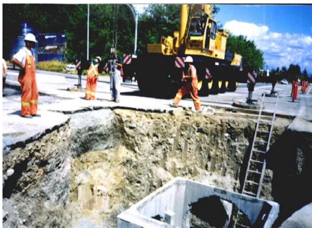
Storm Sewer Installation at 100 Avenue & 154 Street
