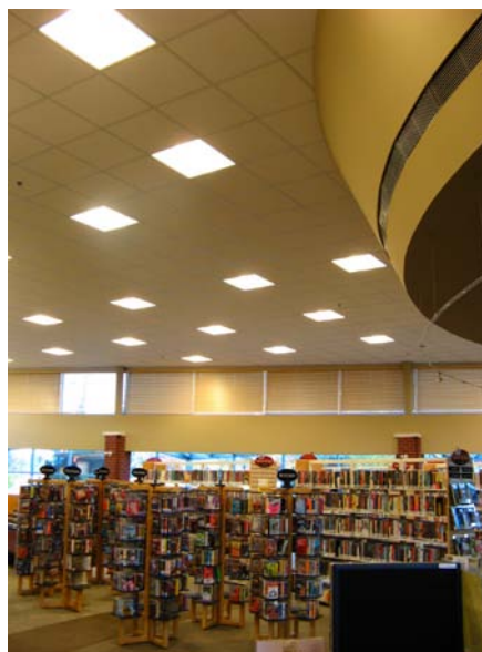
Improved Lighting at Strawberry Hill
