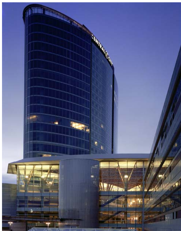
Central City Tower
