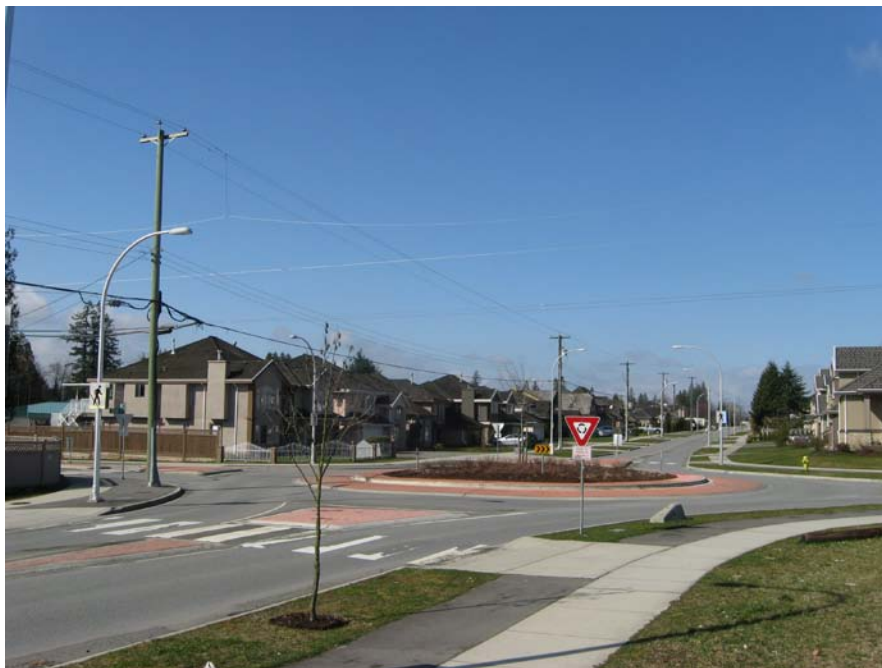
Neighbourhood Roundabout for Traffic Control
