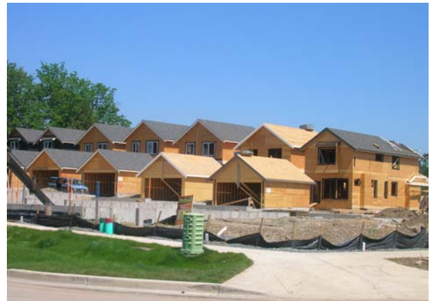
Single Family Dwelling Under Construction
