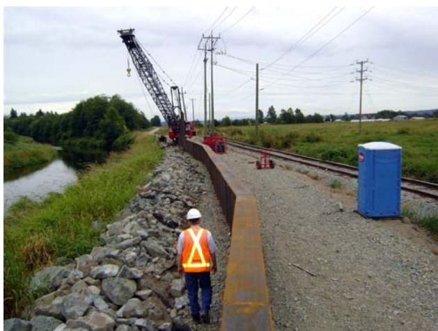
Sheet Pile Wall Construction Along the Serpentine River
