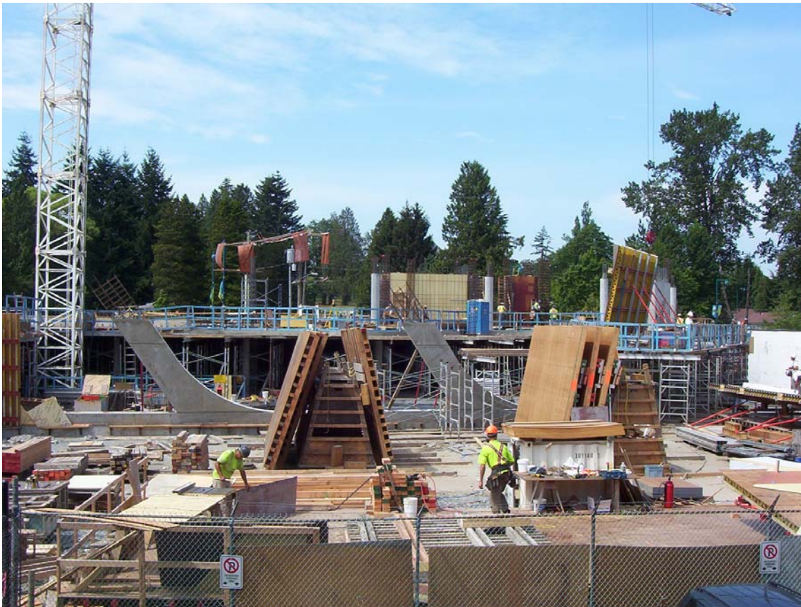
Progress on the new City Centre Library July 2010
