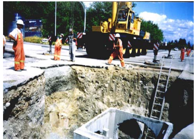
Storm Sewer Installation at 100 Avenue & 154 Street
