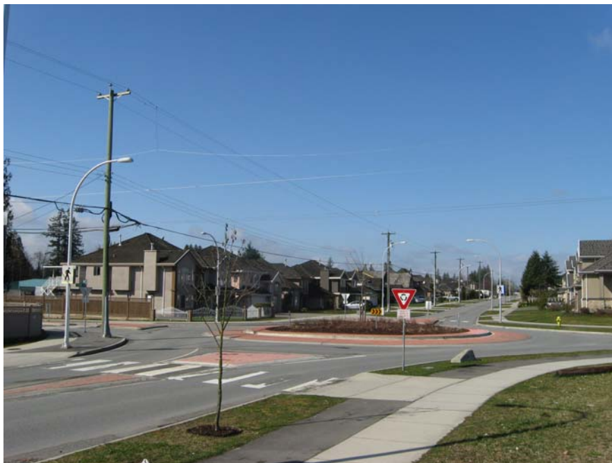
Neighbourhood Roundabout for Traffic Control
