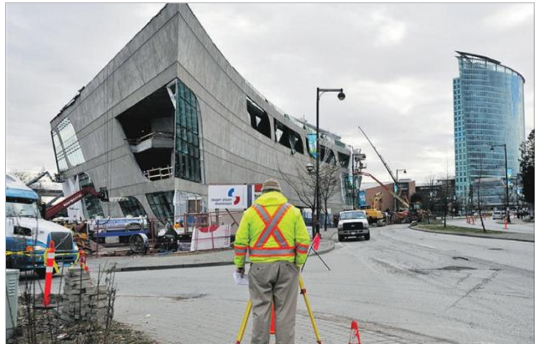
New City Centre Library under construction
