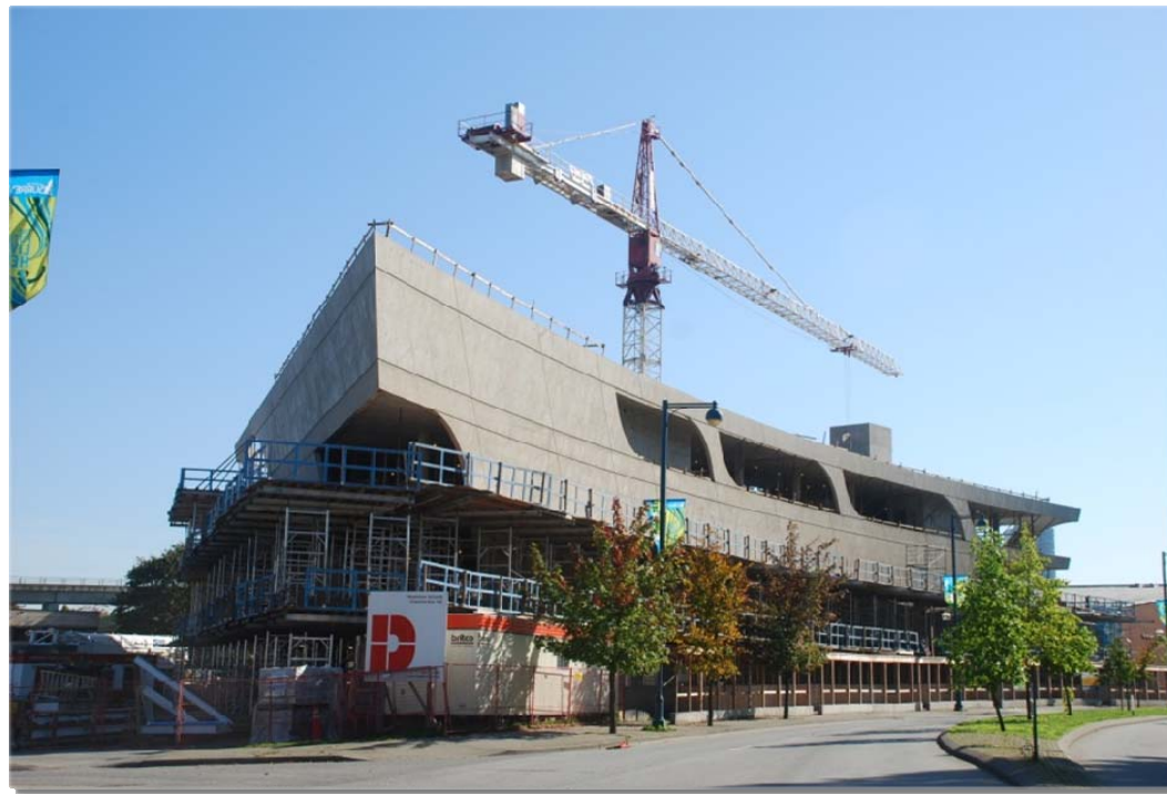
The City Centre Library – construction to be completed Fall 2011
