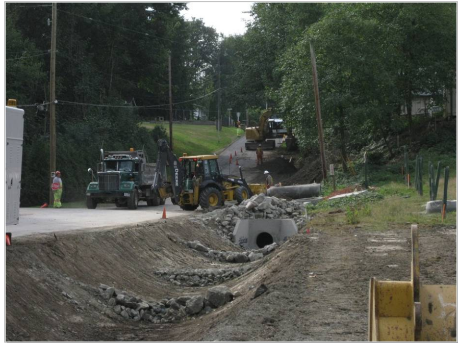
Local Storm Sewer, Outfall and Rock Weir Construction
