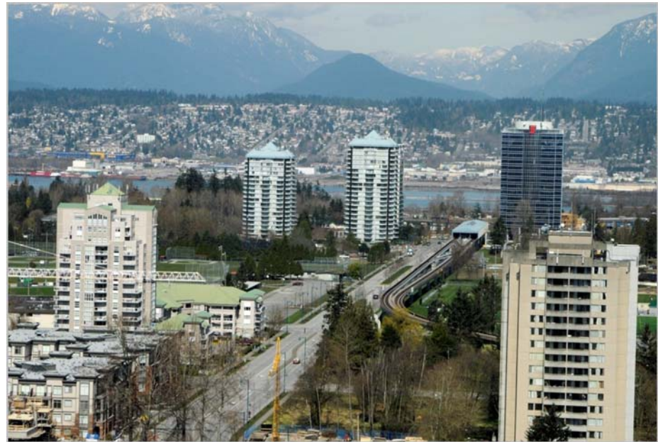
Aerial View of Gateway Skytrain Station in City Centre
