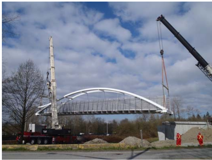
Tynehead Pedestrian Overpass at Highway 1
