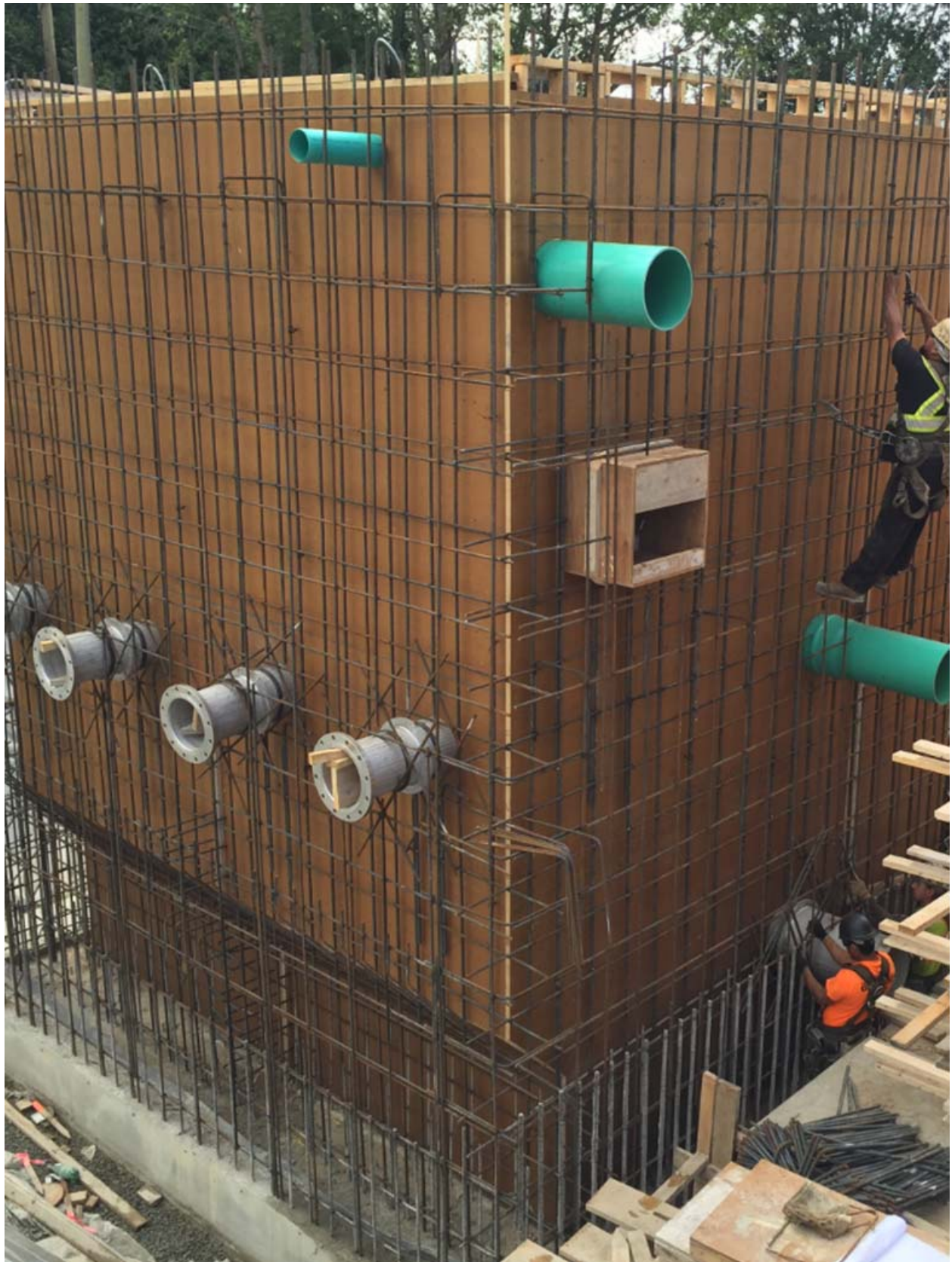
Construction of the Fergus Sanitary Pump Station
