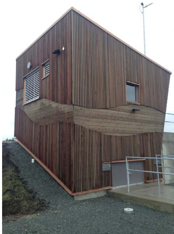
Finlay Pump Station
