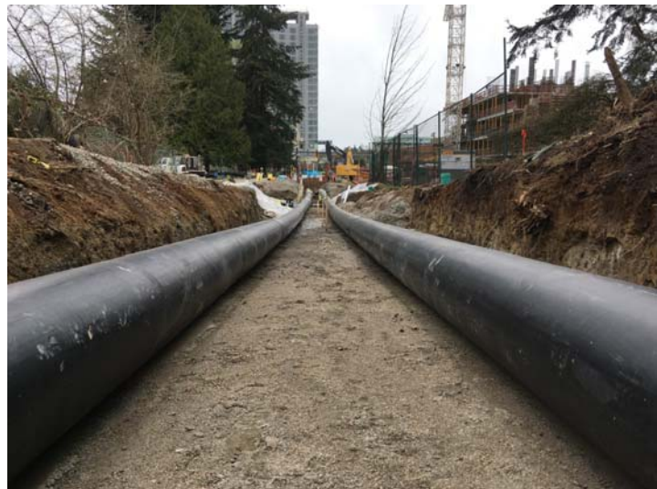
District Energy pipe network expansion under Central Avenue (west of City Parkway)
