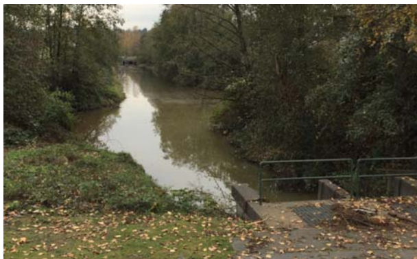
Manson Canal upstream of the Manson Pump Station
