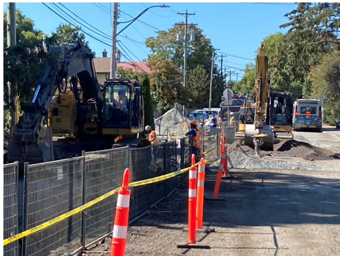
Engineering team on site in Surrey
