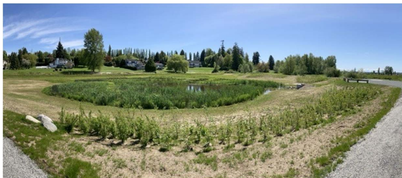
West Clayton Detention Pond (7347 181 Street)
