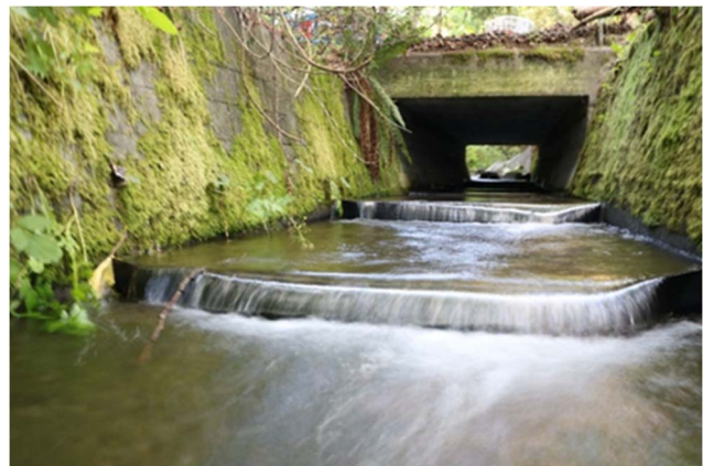
Flexi Baffle Installation on Bon Accord Creek
