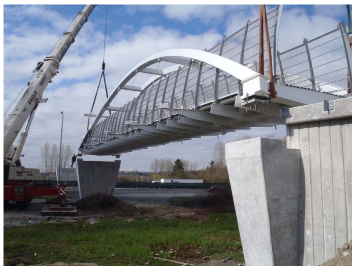
Pedestrian Over cross Construction
