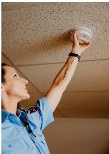
Firefighter checking a smoke alarm
